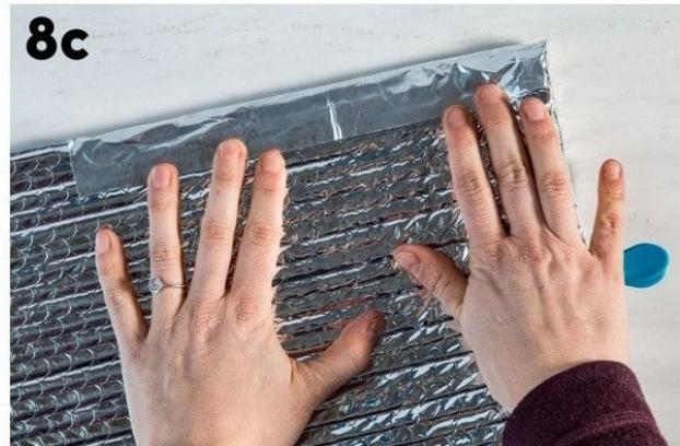
7. Remove the backing from one of the strips of tape. Secure half the width of the tape to a side of the pouch.
